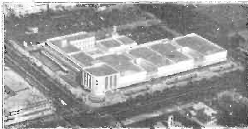
HOLLYWOOD BROADCASTING HOUSE of the N.B.C. where all operating activities are carried out on one floor level. Made possible by the large area of the site, the architectural layout of the four large auditoriums built side by side is strikingly apparent from the air. All roofs are aluminium coated for the reflection of the hot Californian sun rays.
